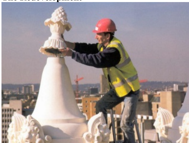
Completion of one of the roof Finials
